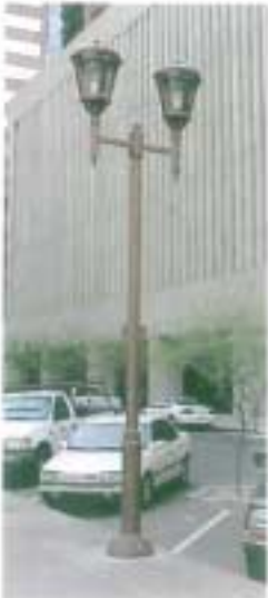
Photo 30. Copper Square streetlight.
