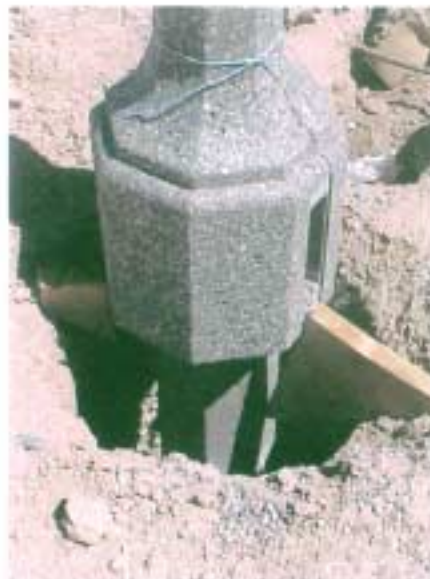
Photo 35. Direct burial base. Concrete poles are available in direct Burial or bolt-down models.
