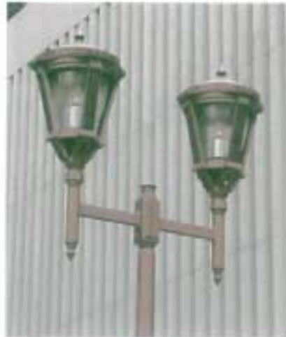
Photo 31. Modern luminaires. Adams Street in Downtown Phoenix.
